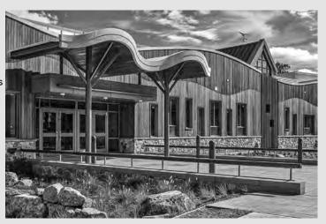
Designed to resemble fingers of an open hand, the classroom wings jut off the back of the building to create protected courtyards. Entire corridors and classrooms can be completely locked down. Hidden gates can secure the property, and perimeter fences are constructed from castconcrete blocks that resemble traditional New England stonewalls.
